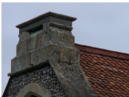
Bellcote, showing concrete copings, and missing top. Tiles to right of picture are slipping
